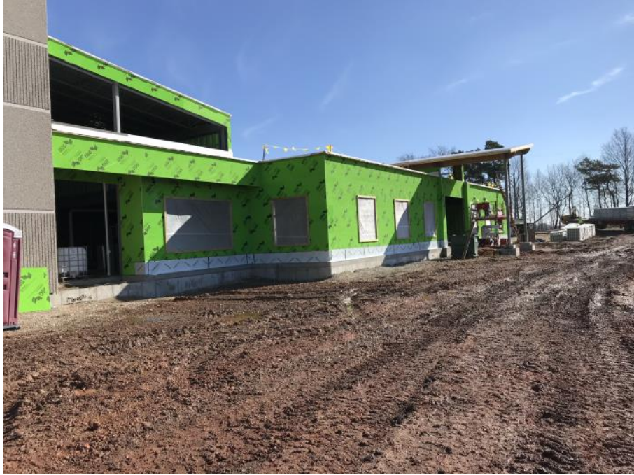
Unit A Office Exterior Studs & Sheathing
