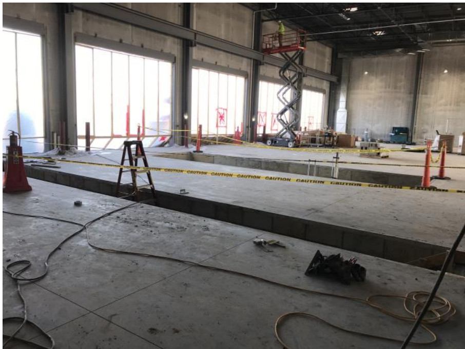
Floors in Unit B Complete
