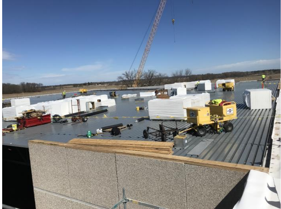
Unit C Roofing Ongoing
