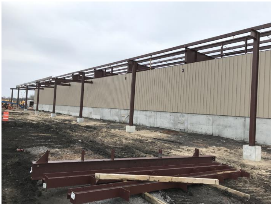
Unit E—Steel Framing and Siding
