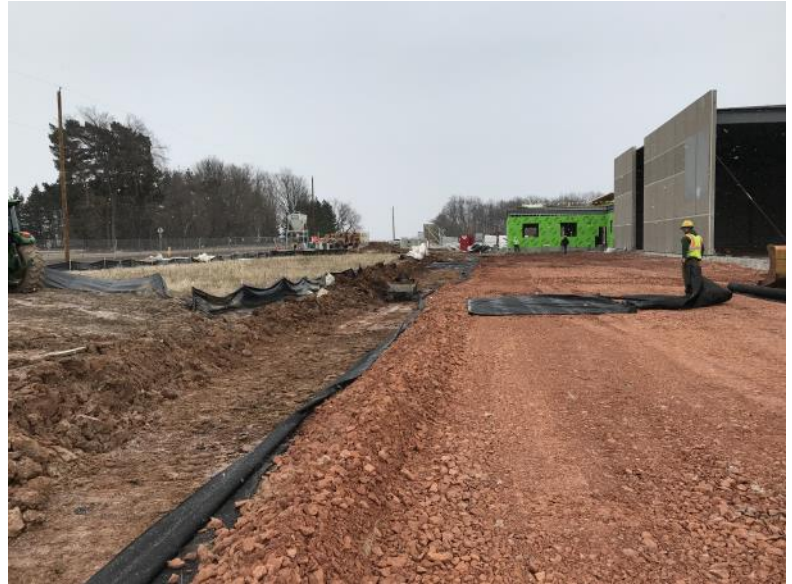
Asphalt Area Subbase-East Side-Unit C
