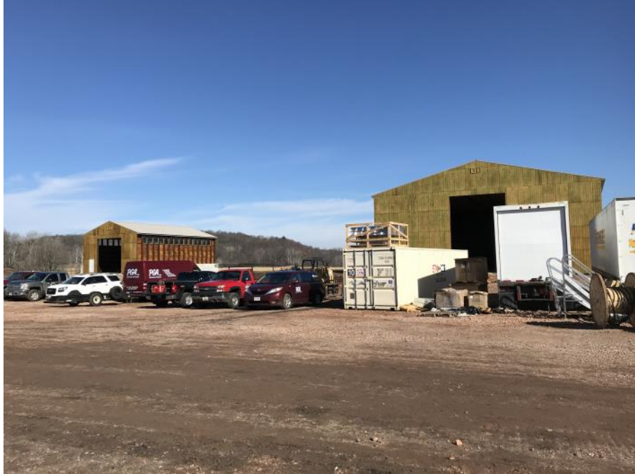
Sand & Salt Shed ready for Overhead Doors
