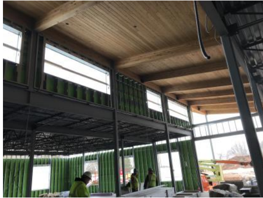
Unit A—Wood Timber and Decking in Place
