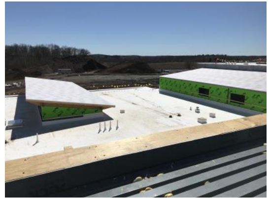
Unit A—Roof Insulation & Membrane—Complete
