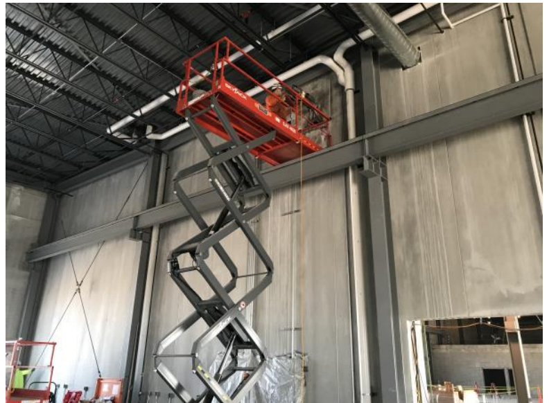
Unit B Sprinklers—Plumbing Rough-ins In Progress
